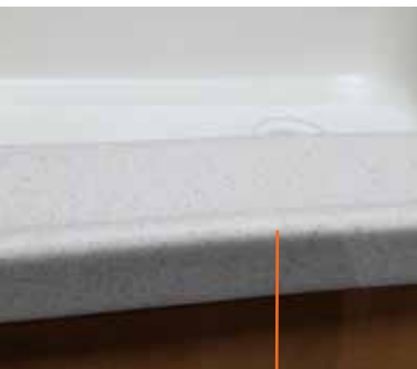
Marine edge counter top minimizes water on floor
