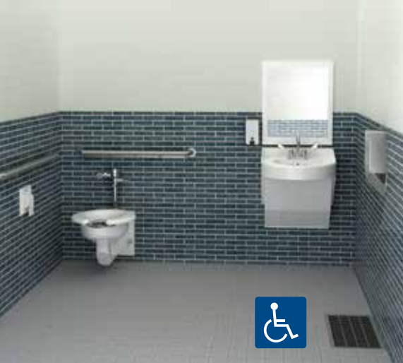
Typical bariatric ADA bathroom featuring an "easy to clean under" bariatric toilet and sink
