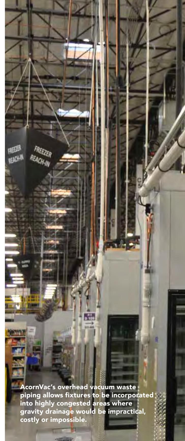
AcornVac's overhead vacuum waste piping allows fixtures to be incorporated into highly congested areas where gravity drainage would be impractical, costly or impossible.
