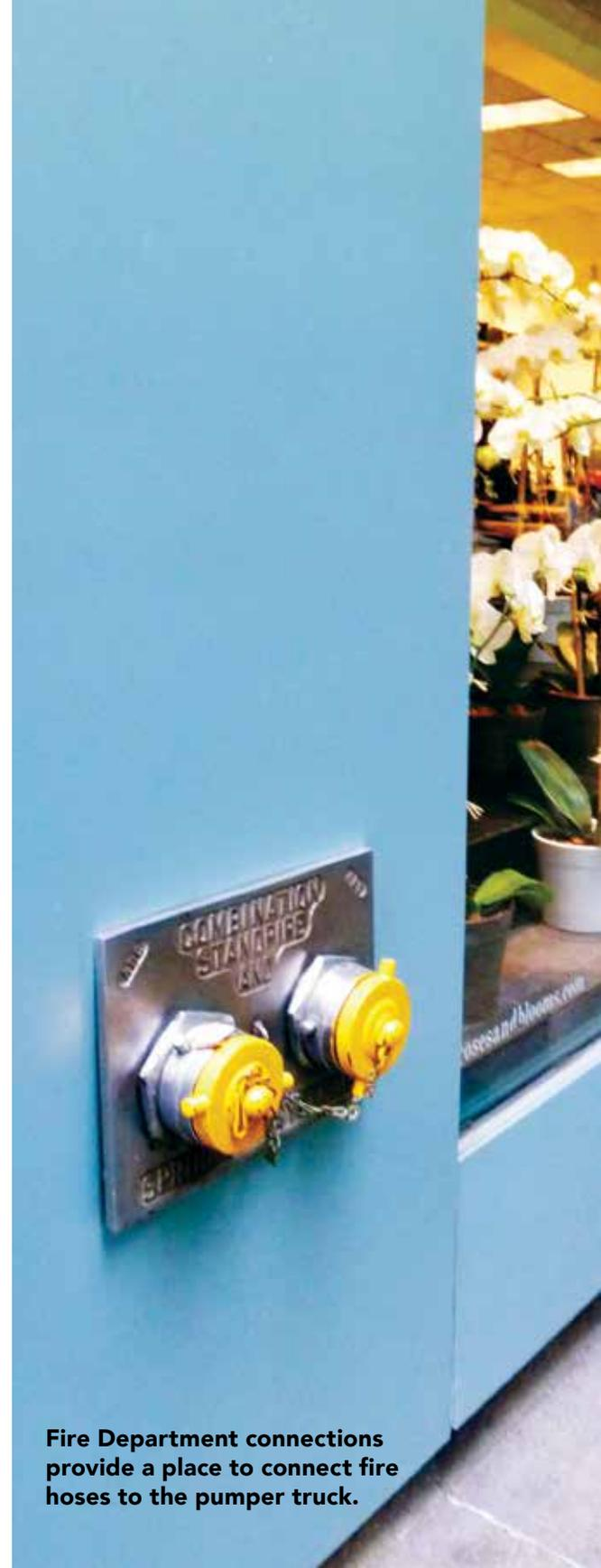
Fire Department connections provide a place to connect fire hoses to the pumper truck.
