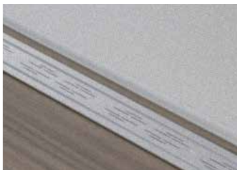
Close up of trench drain
